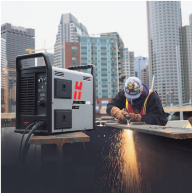
A construction worker uses plasma cutting at a job site.
