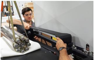
3. Put the attenuator onto the attenuator supports.
