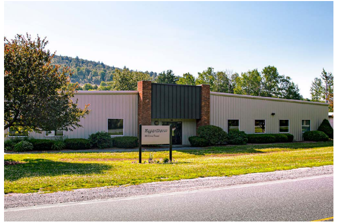
Central manufacturing, 88 Etna Road, Lebanon, NH
