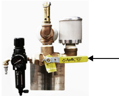
Ball valve in the open position
