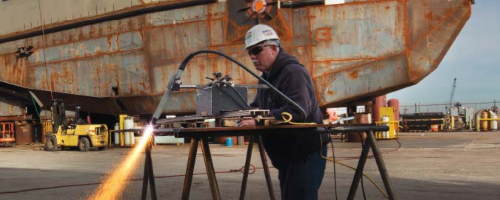
Figure 7. Track burner performing bevel cut on steel plates.
