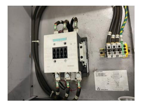
Remove the screws, nuts, and bolts using a Phillips screwdriver, the 13 mm and 17 mm sockets, and the T20 TORX driver. Cut all cable ties.
